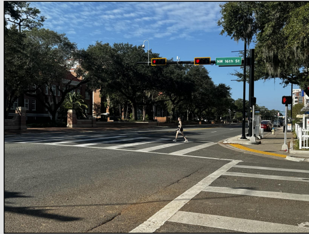
Two New Signalized Intersections
